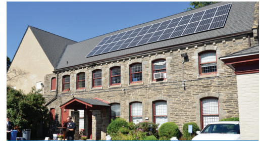
Family Promise of Philadelphia is harnessing solar power to better empower families in crisis.
